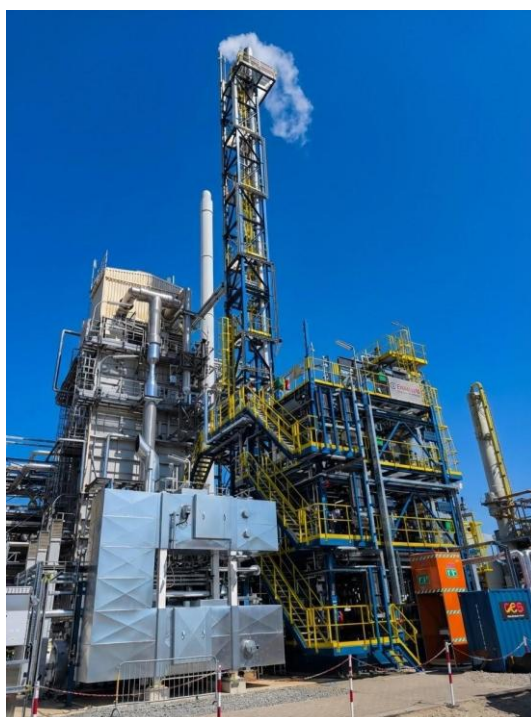
Figure 11: ARCAS - Air Liquide's world's first industrial-scale \text{NH}_3 cracking pilot unit.
